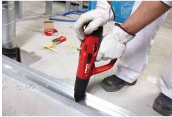
Figure 1: Powder-Actuated Fasteners (PAFs) – an efficient, reliable and safe fastening method.
